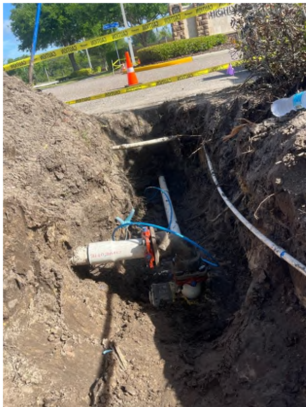
Mainline repair on south side of Clyne Field
