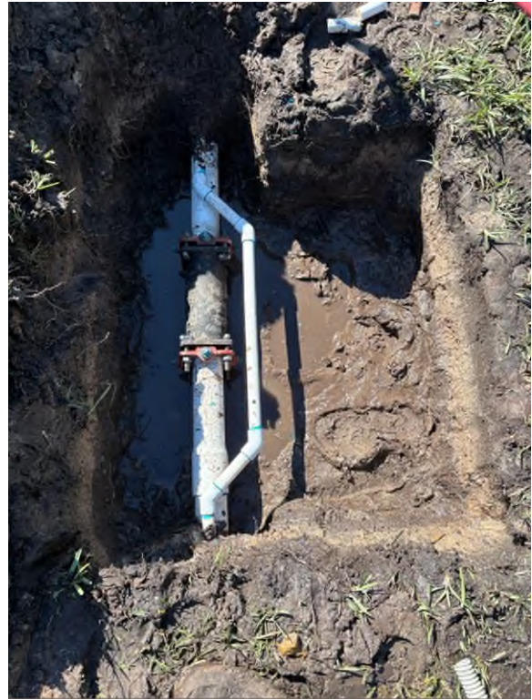
Mainline repair along Ayersworth
